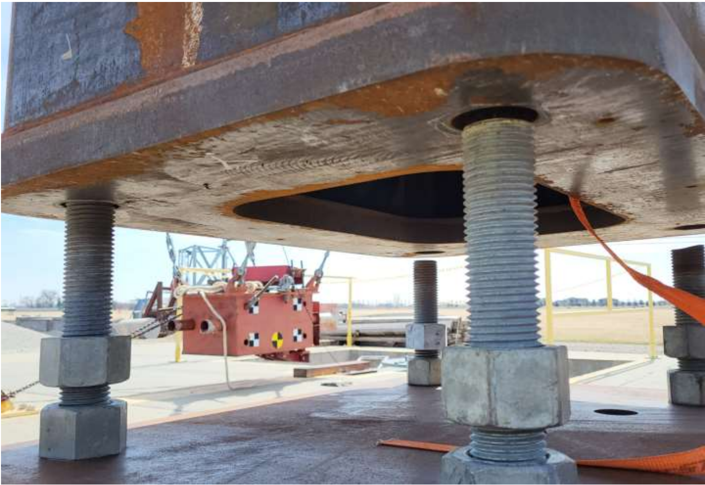
Bottom View of Structure
