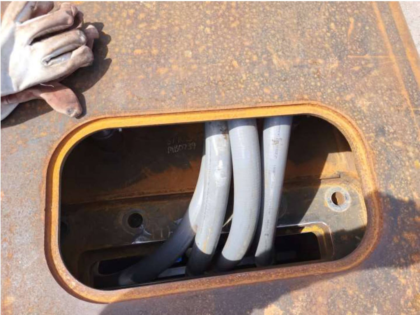
Access at top of Arm
