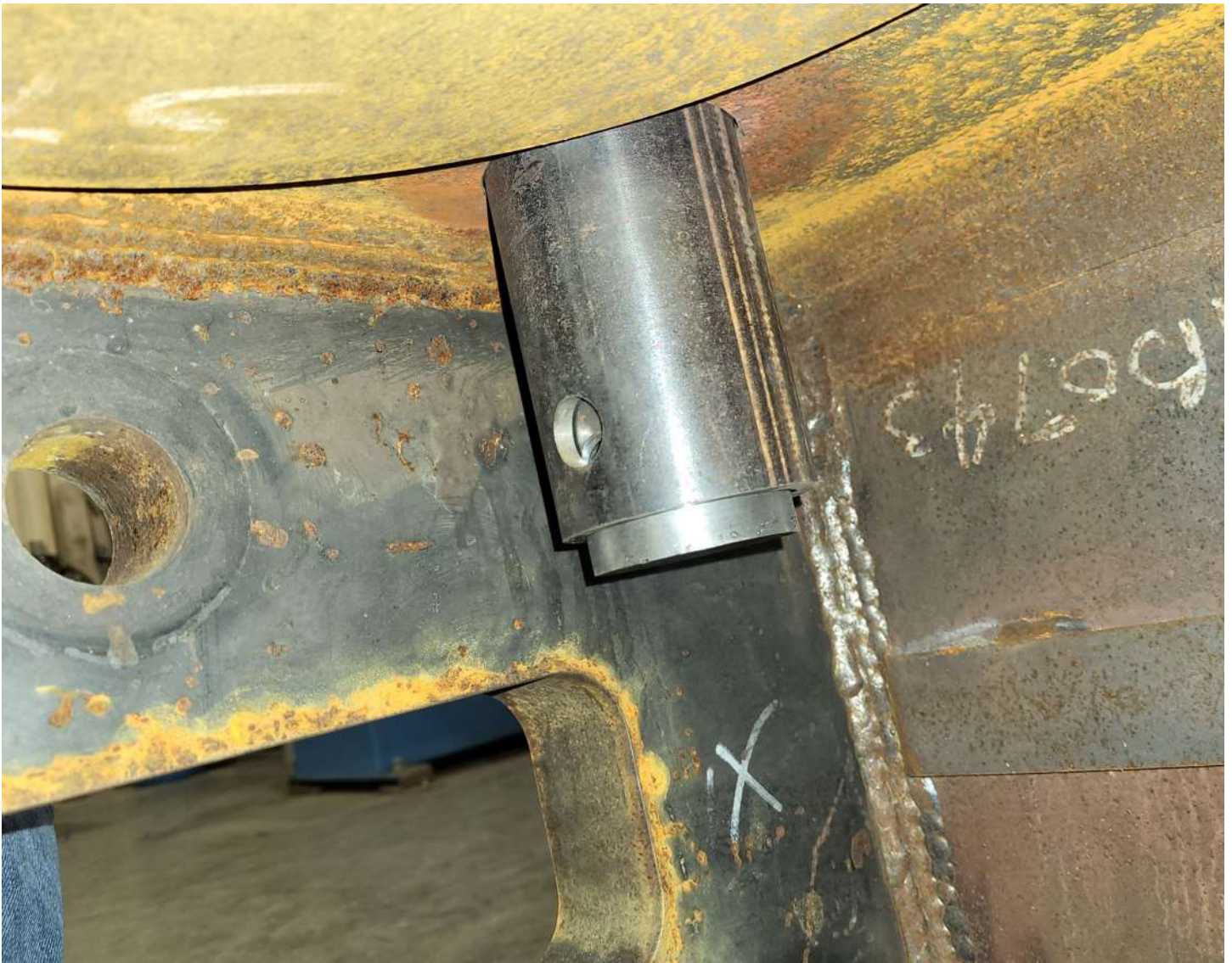
Interior view of Hinge to Pole connection. (Similar connection to a receiver hitch on Pickup truck)
