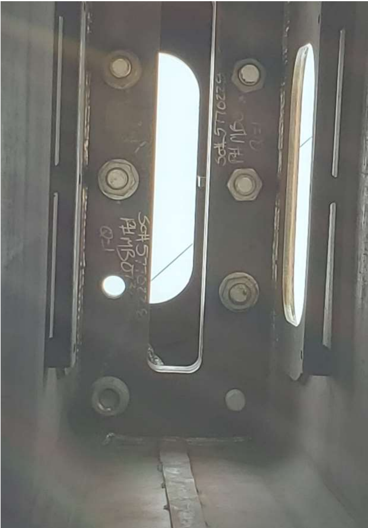
View looking upward at pole to arm connection hardware
