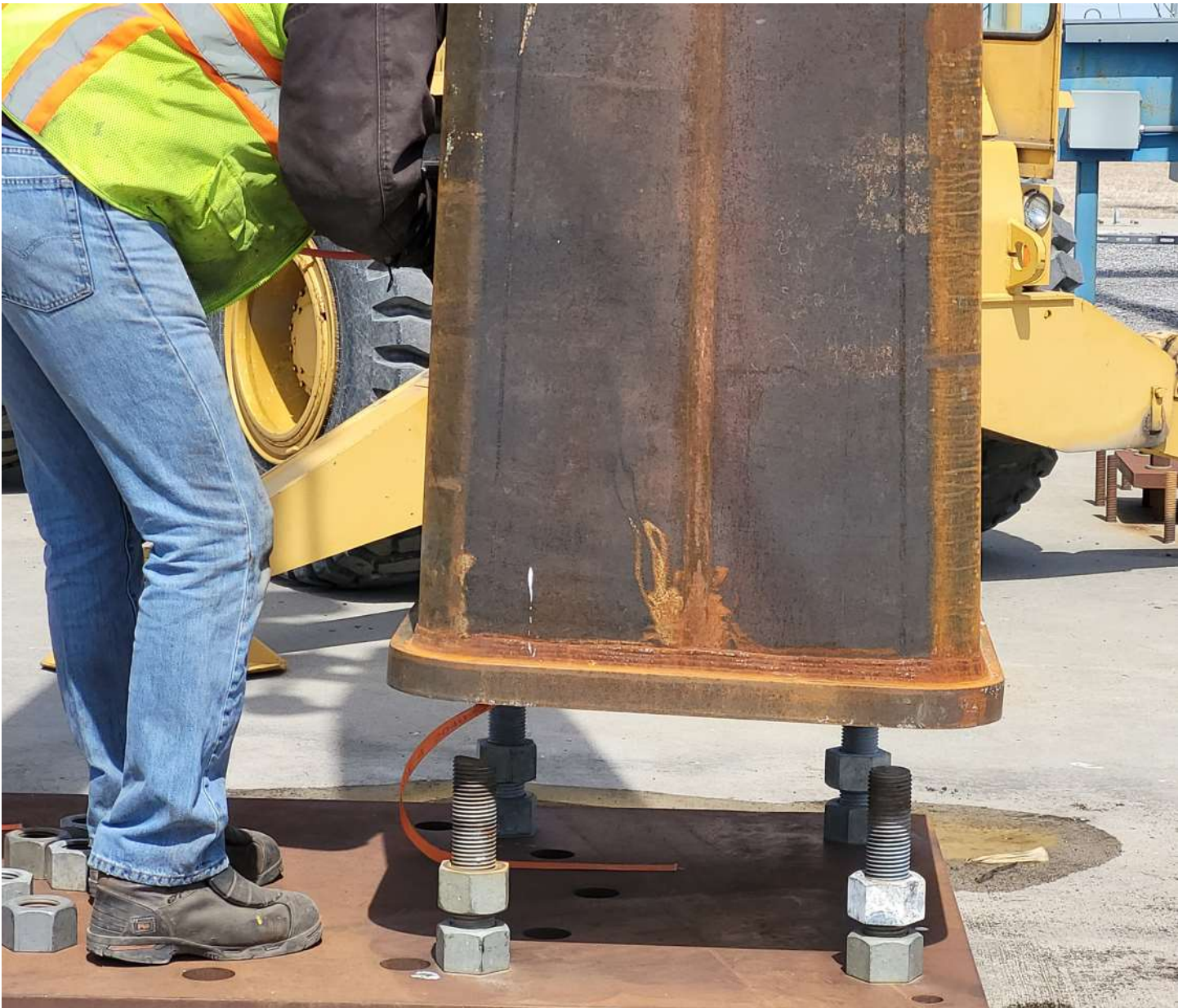
Placing Structure on anchor Bolts
