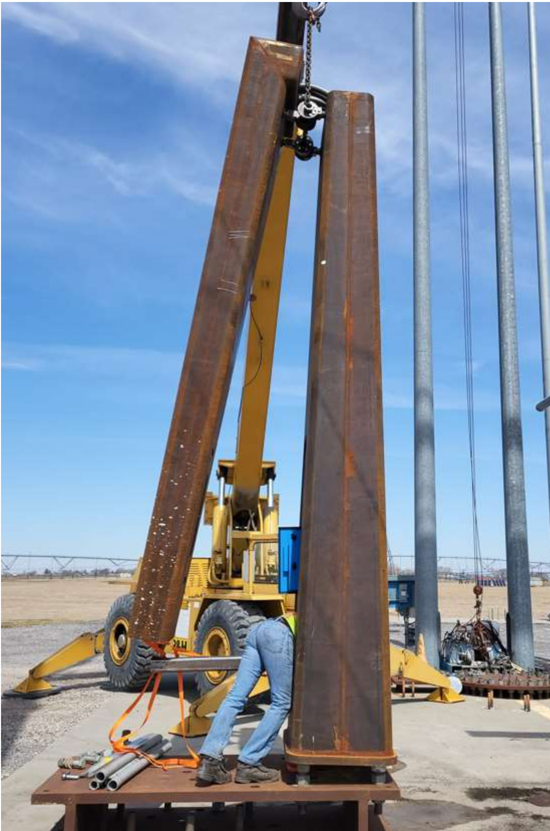
Installation of Anchor Nuts
