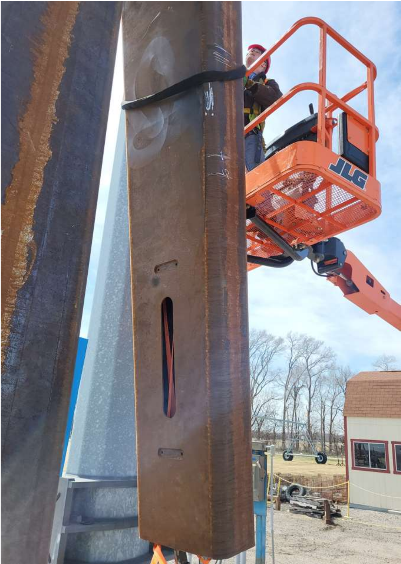
Attachment of sling to arm
