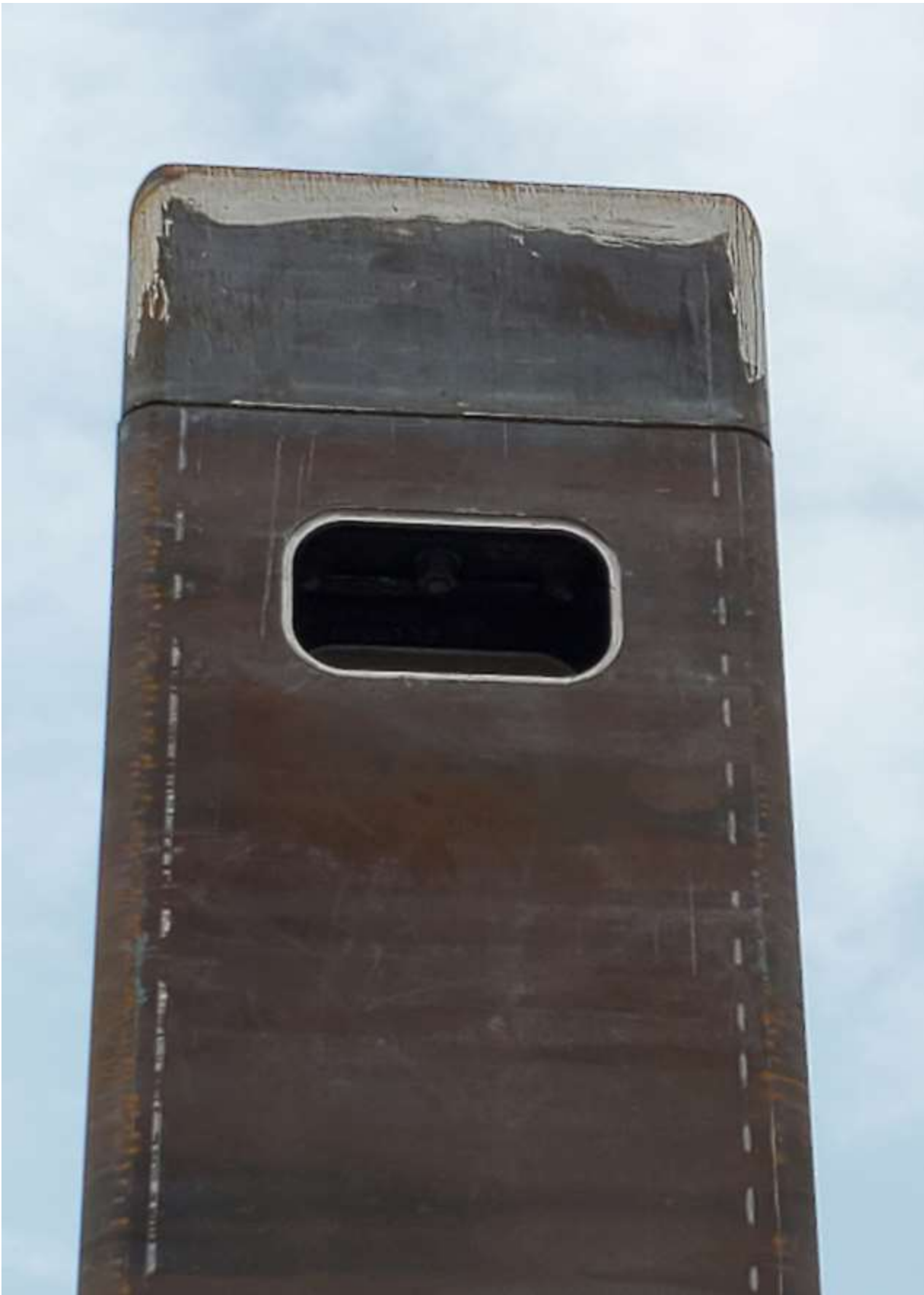
View of Rear of Structure
